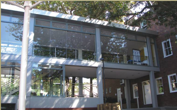
New glass Walkway and Entry
